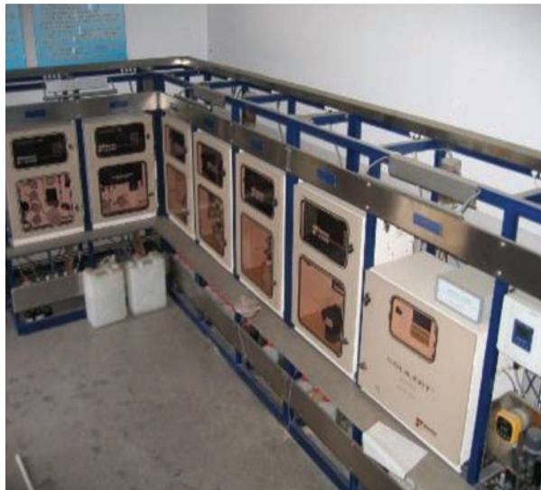
Figure 2: Cabinet analysers at a monitoring station in China.
