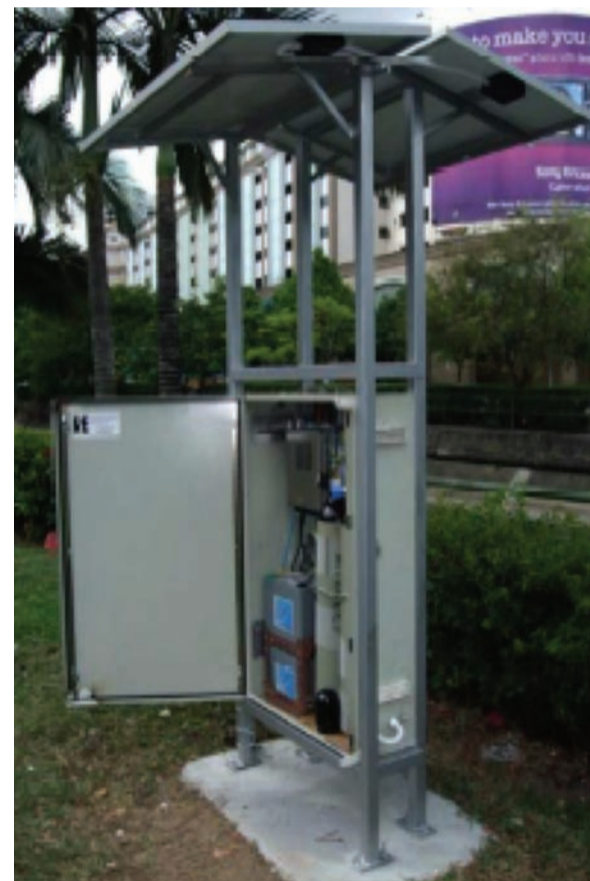
Figure 5: Example of a stand-alone solar powered monitoring station with wireless data transmission to a web-based data collection system as deployed in Singapore.
